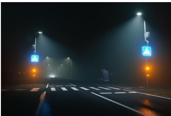
Fig. 5. Operation of the smart pedestrian crossing in reduced visibility conditions
